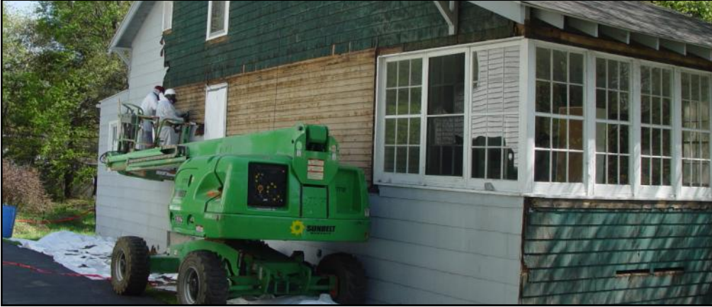
Asbestos abatement on the exterior tile shingles at 320 before demolition permits are issued. All through the month of May, all items of value including furniture and books, decent doors and windows, even copper piping and radiators were removed from 320.
