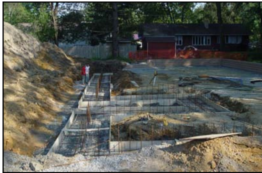
Excavating and Foundation Footings
