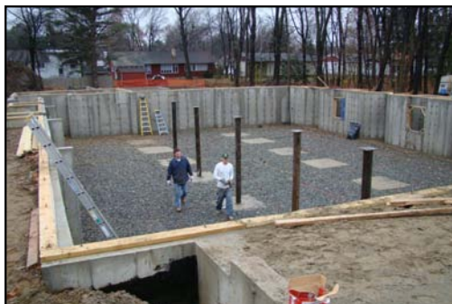
Basement Columns and Start of First-Floor Framing
